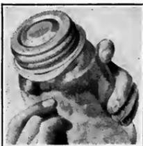
The Cover Should Fit So Tight That the Rubber Cannot Slip Back
